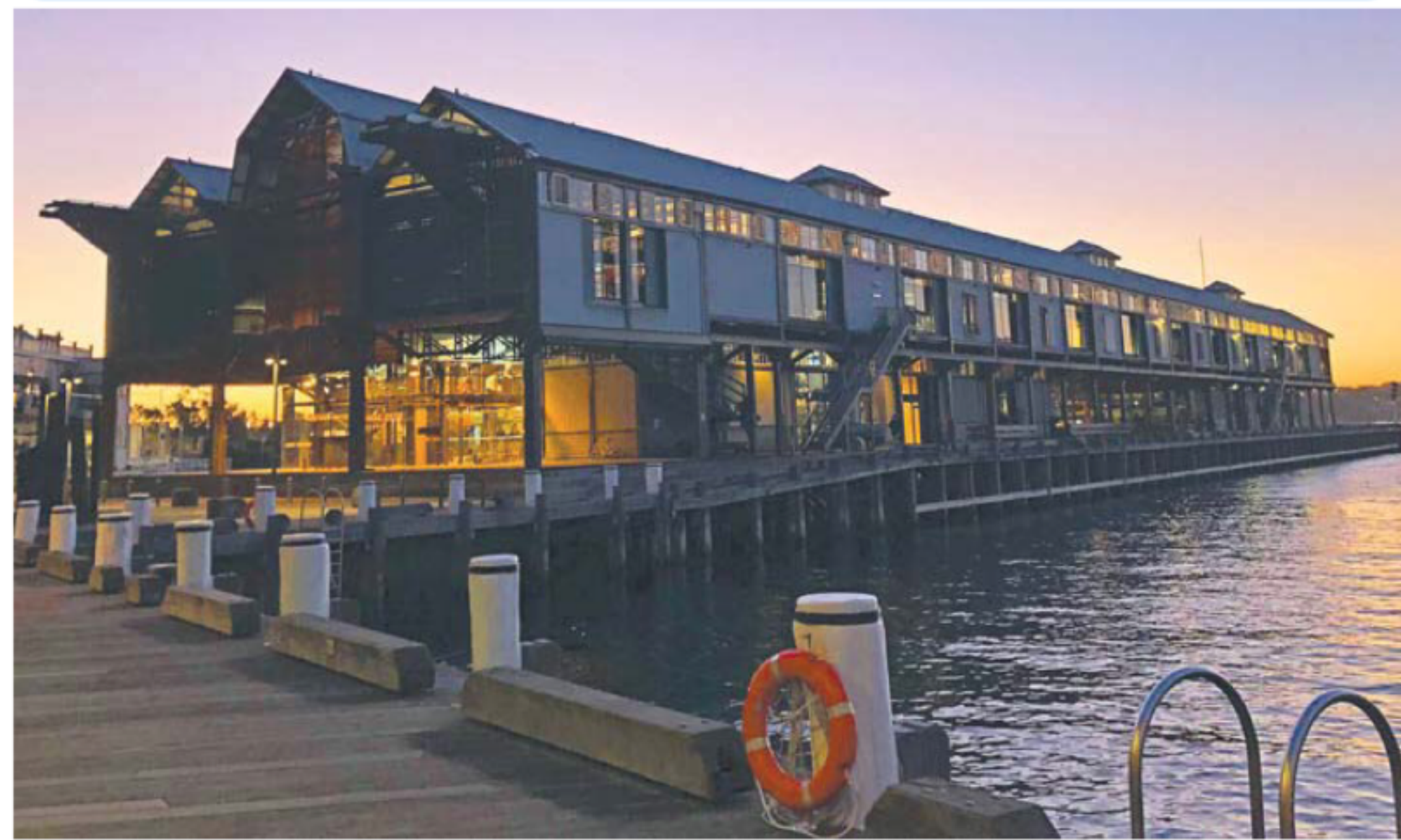
The heritage Walsh Bay buildings at Piers 8 and 9 were rebuilt in 2001 as a quality waterfront office complex
